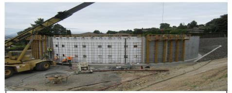
Even before the snow had melted, crews were on site getting prepared to start construction once again. The floor, walls, and column supports for the roof have all been poured. Crews are now currently building the structure to support the forms to pour the roof. We expect the roof to be poured later in June. After additional finish work to be done on the walls and other site work to be completed. Project is estimated to be complete in August!
