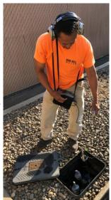
While there is a multitude of ways to help find these leaks, Nob Hill Water decided to try the most straightforward approach first, which is listening to each service connection for a leak. So, since the Fall of 2017, Joel has been out in the system listening for leaks. To date, Joel has found over 200 service line leaks that were not surfacing!
