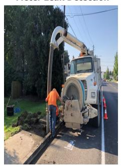
After three years, the meter listening maintenance program is still returning excellent results. By listening to each meter, water leaks that are not surfacing are able to be found. These leaking service lines are then scheduled for replacement. This maintenance program has substantially reduced the amount of lost water over the past three years and has also reduced chlorine and power costs as well.
