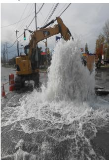
This year Nob Hill Water will replace 20 older hydrants in the water system that were over 60 years old and difficult to operate. Additionally, a concentrated valve exercising program will be staring this fall, targeting pipes that are likely to fail. Nob Hill Water has been using VODA.ai, a machine learning program that lists pipes by their likelihood of failure.
